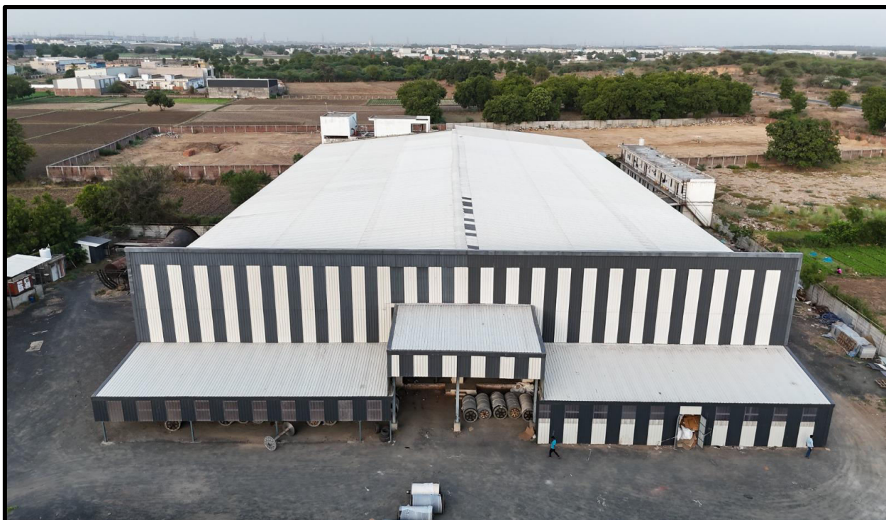
Plot No – 680,681, 683 Opp, Jaganath Industrial Park, Paldi- kankaj, Dascroi, Bareja, Ahmedabad, Gujarat-
